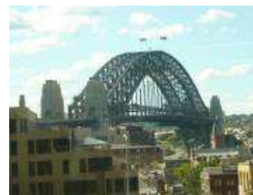
View from Sydney School Lounge
